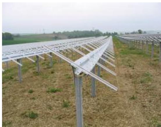
Figure 2: Mounting system for ground based systems
