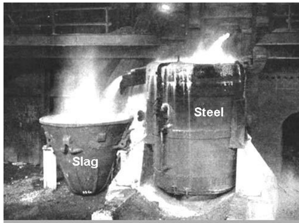
Tapping a Siemens-Martin furnace
