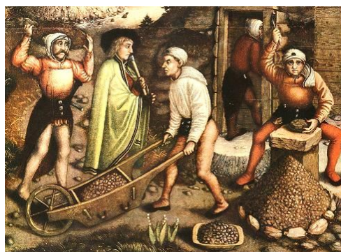
Crushing (silver) ore
