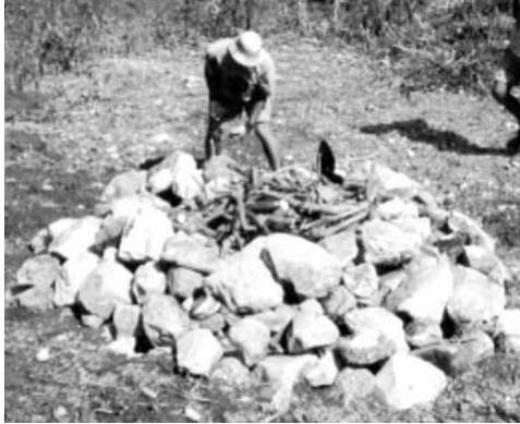
Building a working lime kiln
