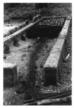
Fig. 9. Stall furnace for the crucible smelting of iron, partly loaded with crucibles packed in coal. Photograph by Dr. Knapp, 1936, in Hunan in province, China.<sup>17</sup>
