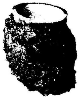
**Fig. 8.** A iron smelting crucible of the Han Dynasty was excavated in Nanyang **m**, Henan **m** province. It was in the shape of a cylinder, but looked like an ellipsoid, as a layer of clay mixed with grass was adhering to its outside surface.<sup>6</sup>
