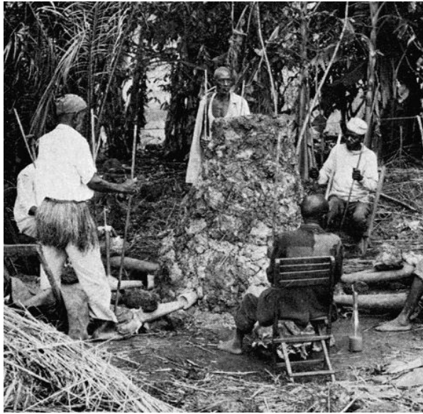
Haya smelter in 1977. Note the 8 (leaky) tuyeres!
