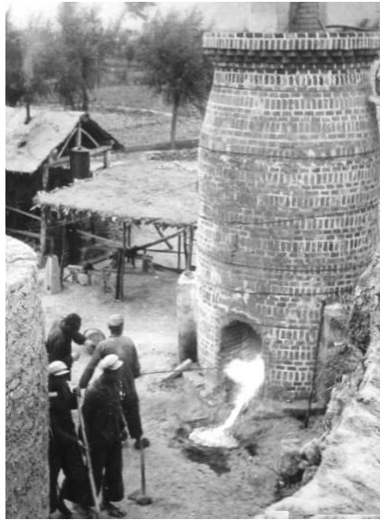
Tapping of a blast furnace in Wushan, Gansu, 1958
