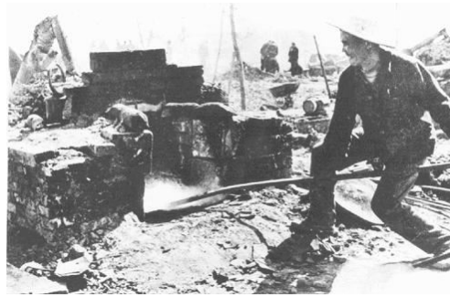
Puddling steel around 1958 "Operation of a traditional type of fining hearth in Shanxi"
